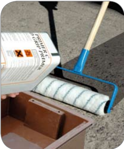
Use Primer C on absorbent surfaces
