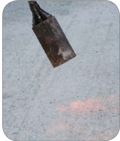
Drying with a hot air lance
