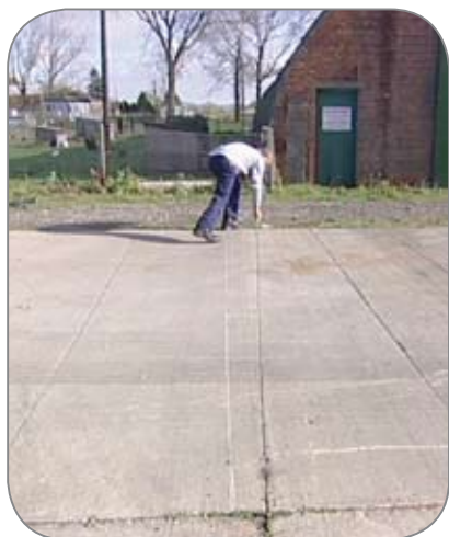
Concrete slab joints
