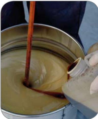
Add the activator slowly whilst mixing
