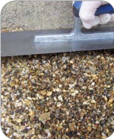
Compress, level and consolidate with a bullnose trowel
