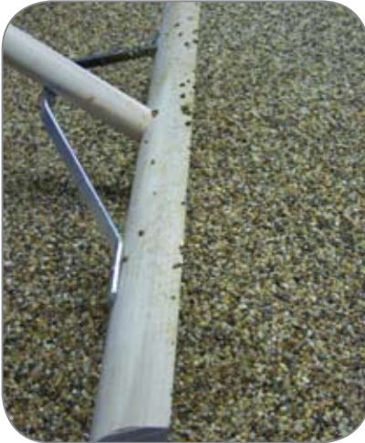
Pre-level using a rake or a flat-bladed squeegee
