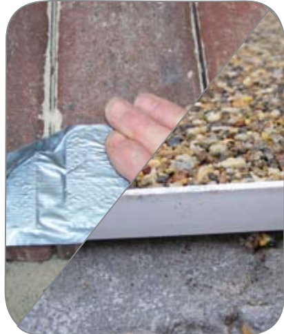
Masking-off with peelable tape & end-stop beading
