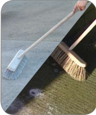
Brushing the surface and removing contamination
