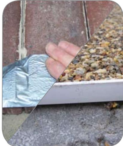
Masking-off with peelable tape & end-stop beading
