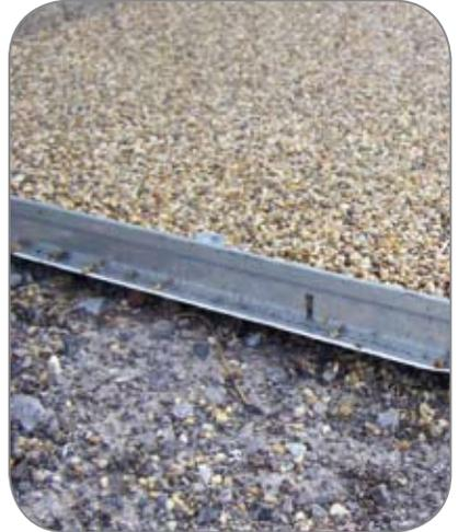
Work to battens or end-stop beading where required
